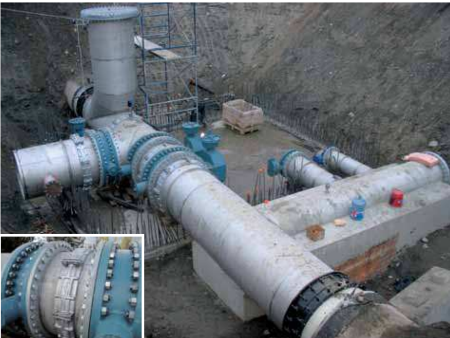
24" (600mm), 36" (900mm) and 48" (1200mm) Model R-88 Couplings with stainless steel rings used on stainless steel hydro electric pipe line, Vernon, British Columbia, Canada
